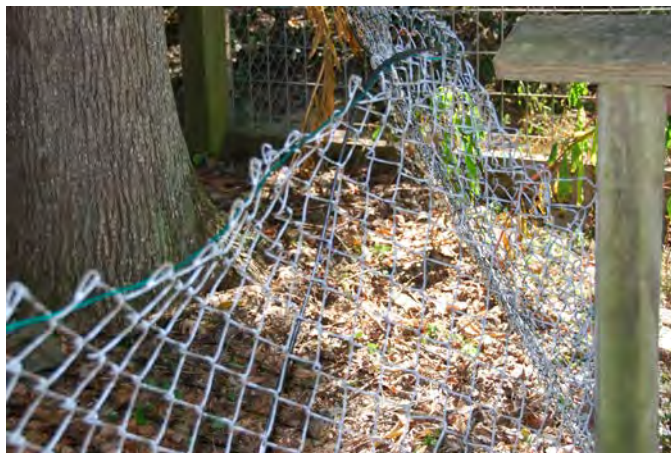
A bent, sagging fence next to a tiger cage at Catoctin Zoo could easily allow a child to penetrate the public safety barrier.
