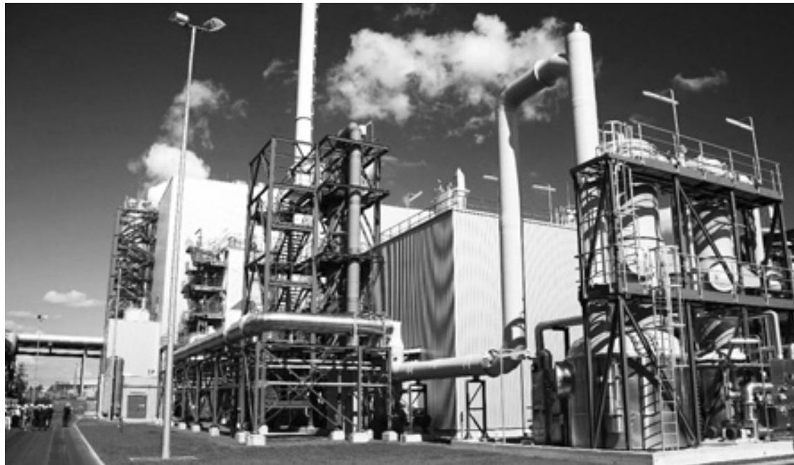
Cryogenic storage stores power provided by renewable energy sources or off-peak generation by chilling air into liquid from minus 190 degrees Centigrade. It is then stored in an insulated tank, and then allowed to warm up at a later time, to expand it and drive a turbine to produce electricity.
