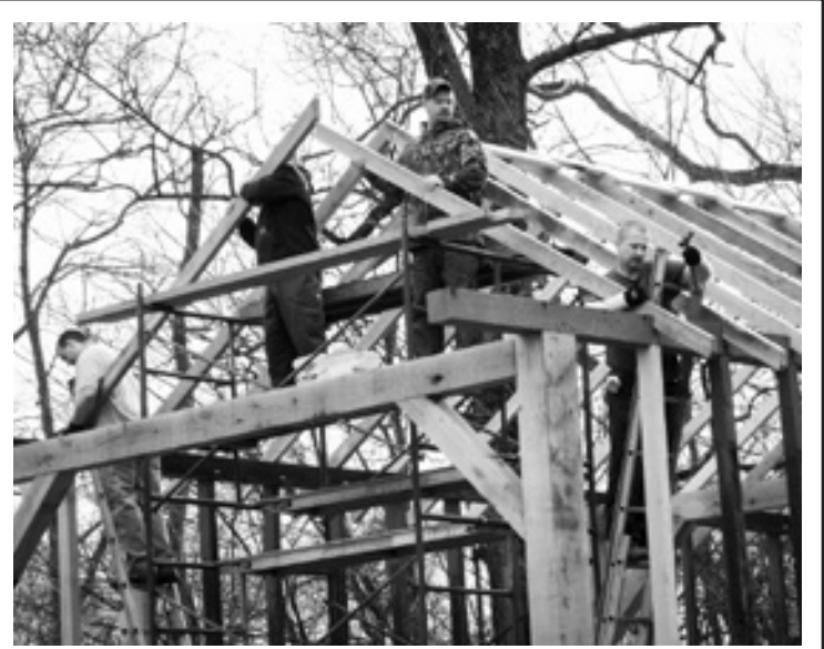
Repair work on Roddy Road covered bridge
